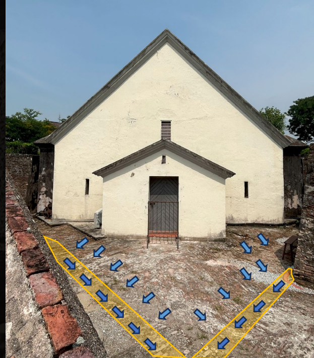
Figure 18: Runoff water management system within the bastion. Figure by author, 2025.
