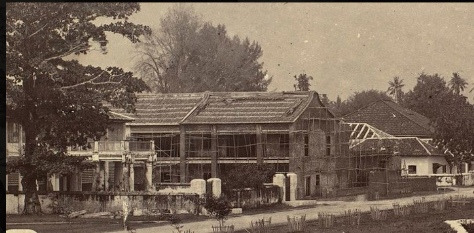
Figure 21: Construction of a shophouse in Penang. Wooden scaffolding and plastering of exterior surfaces.
