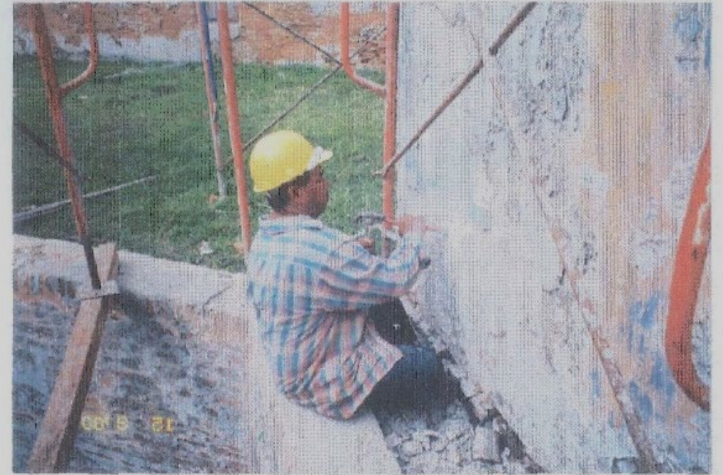
Figure 22: Removal of plaster during the 2000 Restoration campaign. Figure by Ghafar, 2000.
